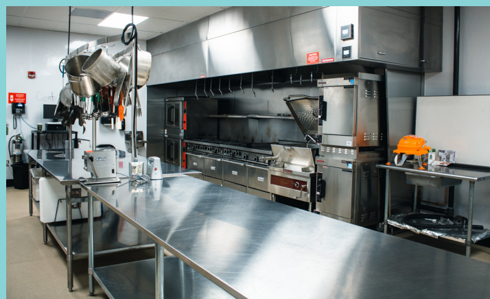
Newly remodeled kitchen at the Montgomery County Job Center
